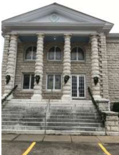
Before the repairs to our church
