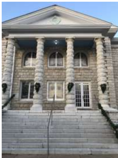
After the repairs were done
